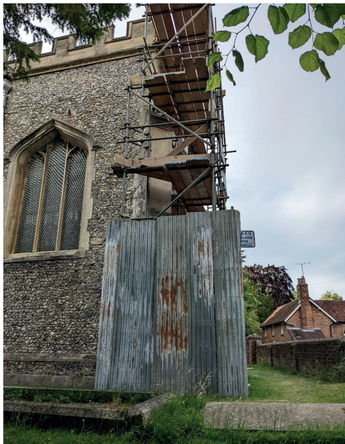
Scaffolding erected to facilitate inspections and repairs of stonework
